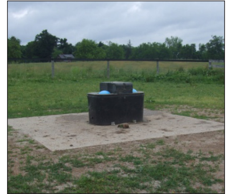
Figure 2. The stability and wear of a watering pad area treated with soil cement two years prior.
