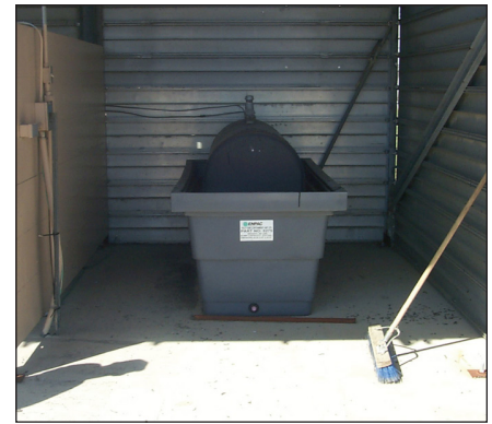
Figure 3. A separate area used for storing fuel (diesel) for the incinerator.
