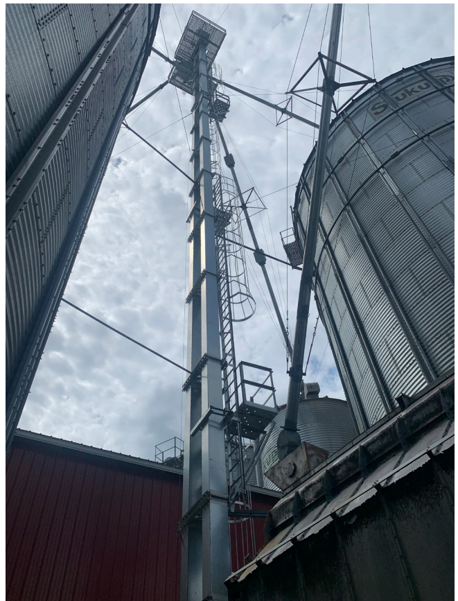
Image 11.5. Grain legs must be tall enough to provide proper angles to allow grain to fall into bins by gravity.
