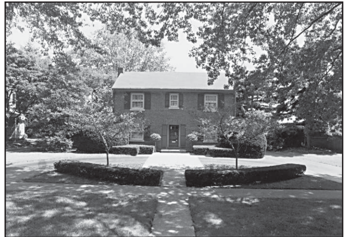
Figure 18a. The extension of this entrance foyer into the front yard creates an entrance courtyard.
