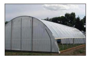
The frames, which can be constructed of metal pipe, wood, or PVC pipe, are covered with one or two layers of greenhouse-grade polyethylene; those covered with two layers of plastic have an air layer in between, thus offering better insulation and, consequently, more cold protection.
