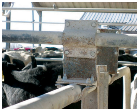
Figure 17. An example of a welded pipe fixture used to raise the height of a neck rail.
