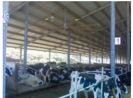
Figure 25. The ideal freestall barn maximizes natural ventilation with high, open sidewalls and a ridge vent opening and supplements natural ventilation with fans used to increase air flow and exchange.
