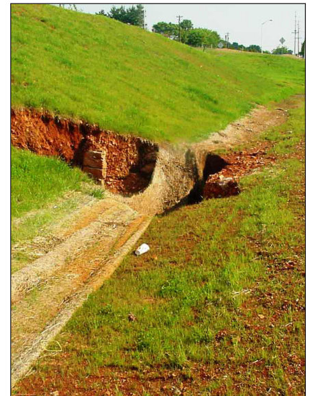
Figure 4. Water was channeled into this sinkhole, causing it to grow deeper and wider.
