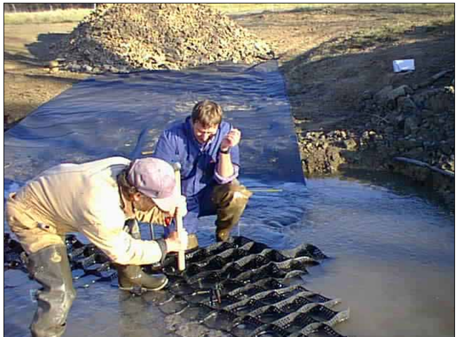
Figure 7. Geoweb, when placed over geotextile, offers extra stability for streams with soft beds.
