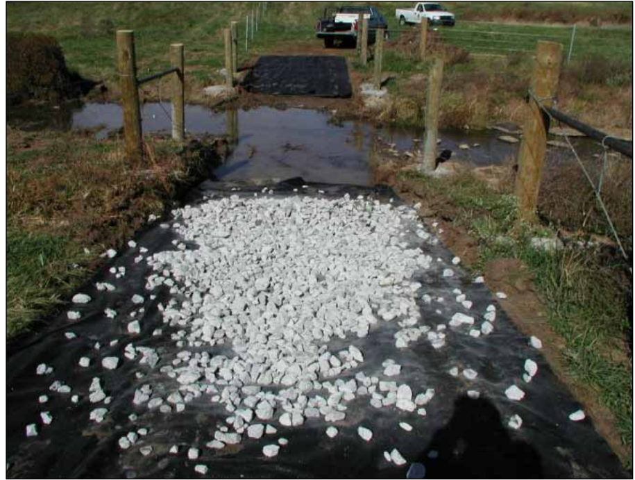
Figure 4. After anchoring the geotextile fabric, place and compact a 6-inch base layer of large aggregate.
