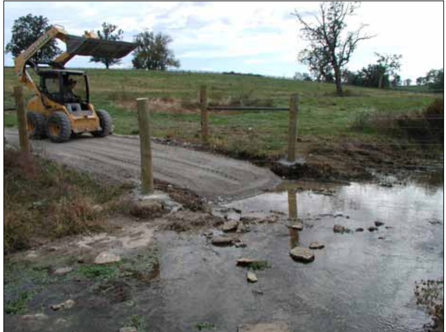
Figure 6. A 4-inch layer of dense grade aggregate (DGA) is placed over the base layer and compacted to form a smooth surface.
