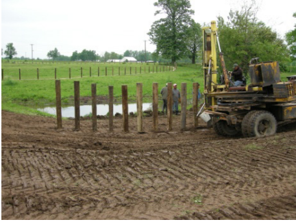
Figure 6. Posts are installed to support the bank in a grade stabilization structure.
