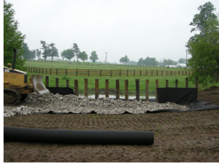
Figure 7. The posts are reinforced with geotextile fabric and rocks, which form a base for the soil.
