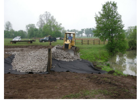
Figure 8. Rocks are pushed up on both sides of the posts to collect soil runoff and filter water before it reaches the stream. Rocks also give newly established vegetation something to cling to.
