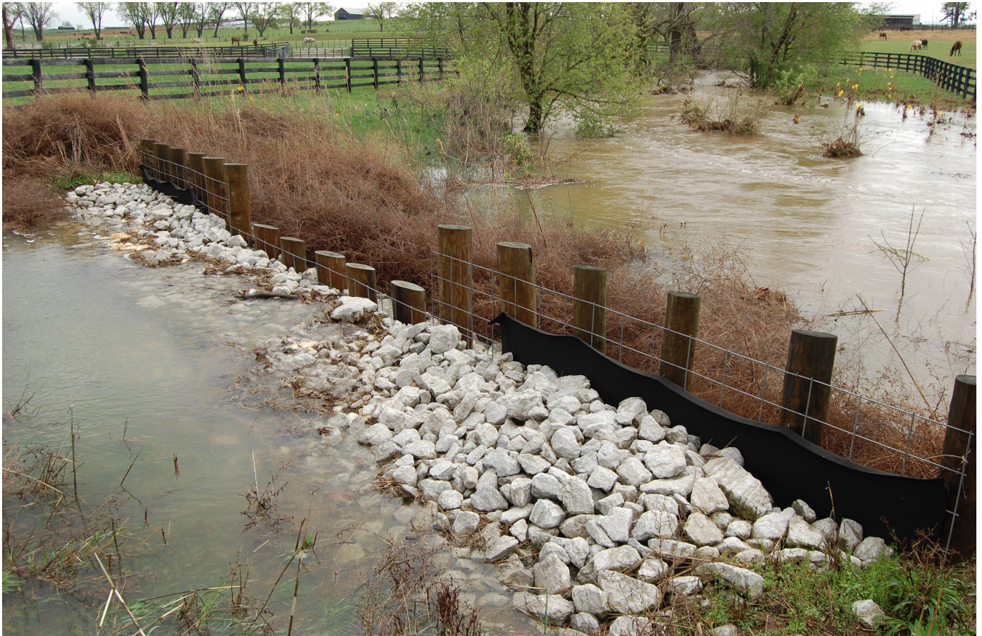
Figure 9. The completed grade stabilization structure prevents erosion by controlling the flow of water, absorbing stream energy, and controlling the elevation change.
