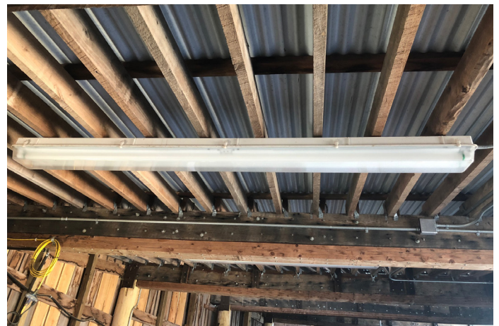
Light coverings prevent shattered bulbs from getting into your product.
