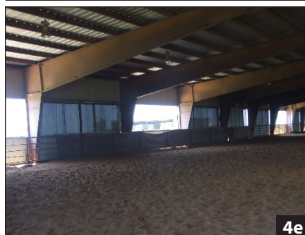
Figure 4. End wall door for equipment access to the indoor arena (a); knee wall around the indoor riding arena (b); wall separating the riding space and observation area (c); a wood framed indoor arena (d); and a steel framed indoor arena (e)
