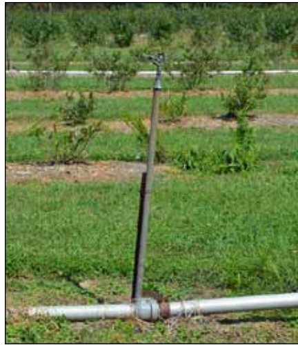
Figure 6-3. Overhead irrigation consists of nozzles mounted onto risers.
