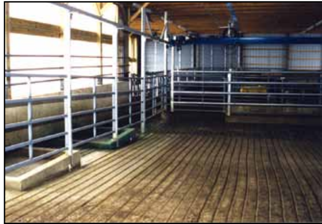
Grooved concrete floors and scored rubber padding improve footing and comfort. This is most important for high traffic areas such as parlor holding pens and feedbunk alleys.
