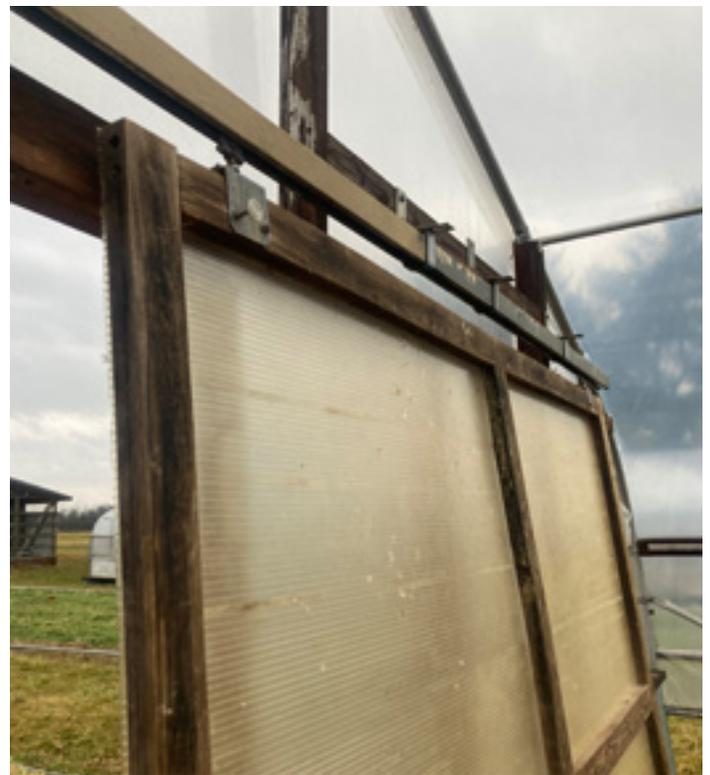
Figure 12.6 Sliding door hardware.
