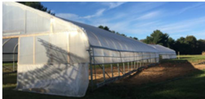
**Figure 12.4** Windstorm-shifted tunnel. Windstorms moved tunnels when anchors had not been fully installed. Note the structure has been picked up and moved diagonally in the plot.
