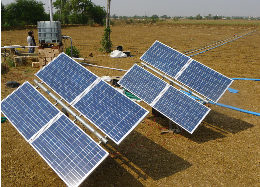
Figure 5. One-acre field in Gujarat, India, irrigated using a combination of a 1 hp solar-powered DC pump and ultra-low pressure drip from a gravity tank (background); system pressure was 2-3.5 psi.
