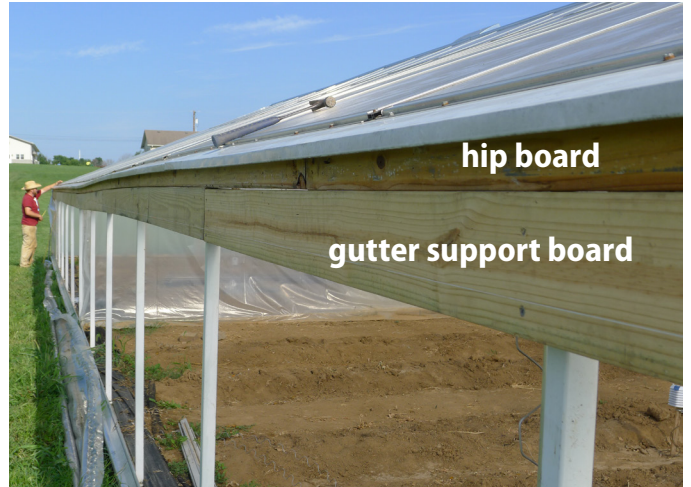
Figure 8. Hip board and gutter support board.
