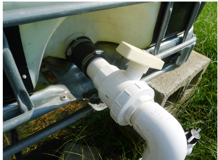
Figure 21. A main shut-off valve is required at the tank outlet.
