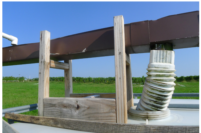
Figure 14. Simple gutter support structure made from treated pine.
