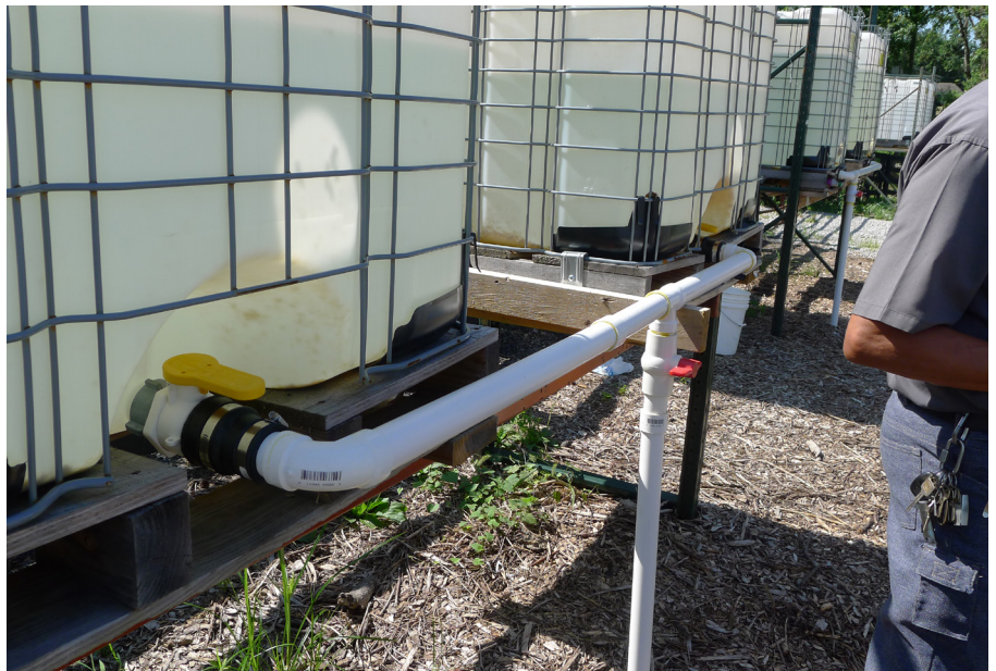
Figure 15. 1½-inch outlet fitting designed for a 275-gallon tote tank.
