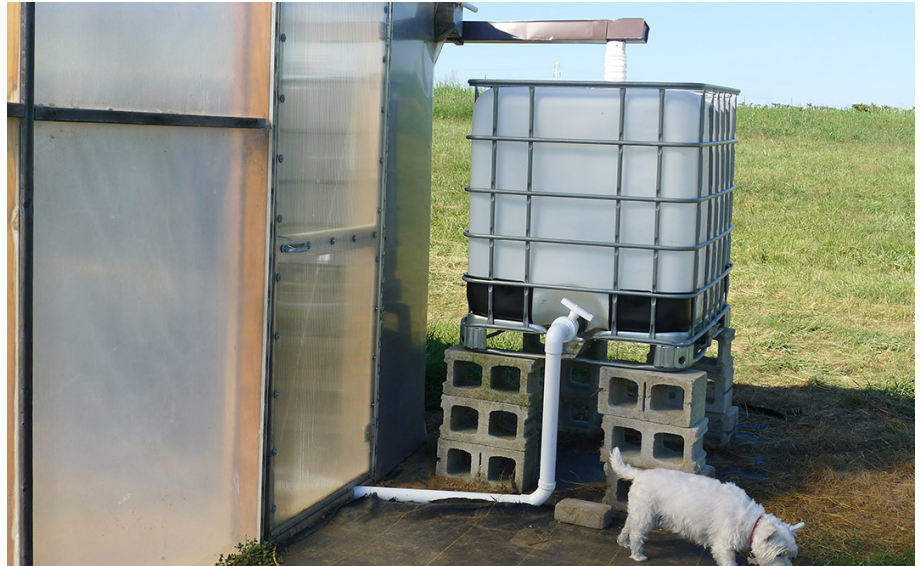
Figure 3. A low tank used to irrigate a small high tunnel with rainwater.
