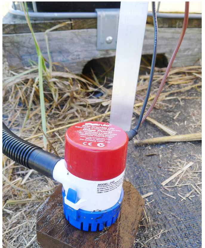
Figures 25a and 25b. Small 12-volt, 2 amp DC bilge pump used with a 12 volt battery and solar panel. The pump is attached to a scrap of Hardie™ board cut to fit inside the tank opening. Flexible marine bilge pump tubing is used as the pump's delivery pipe.
