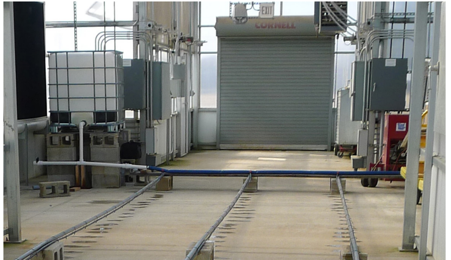
Figure 4. Test setup for measuring uniformity of watering from drip irrigation with only 1 psi system pressure.
