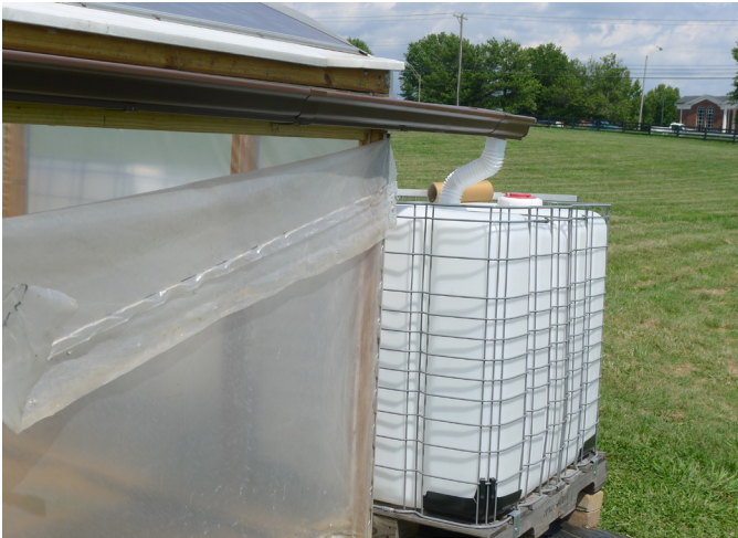
Figure 7. While seamless gutters are preferred, sectional gutters sold in home improvement stores can also be used.
