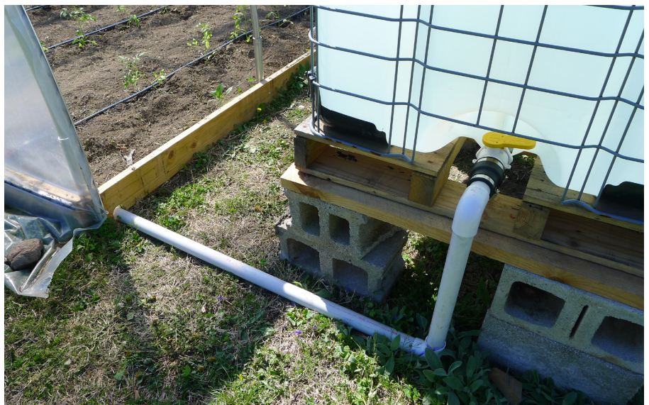
Figures 16a and 16b. Tote tanks with ball valves fitted to PVC pipe with Fernco™ couplings.
