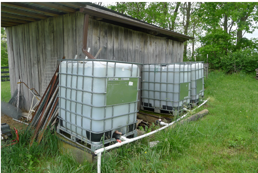
Figure 6. Three “tote” tanks joined together to collect rainwater from a small outbuilding in Wilmore, Ky. The tanks have a total capacity of 825 gallons and are used to irrigate an adjacent vegetable garden and high tunnel.
