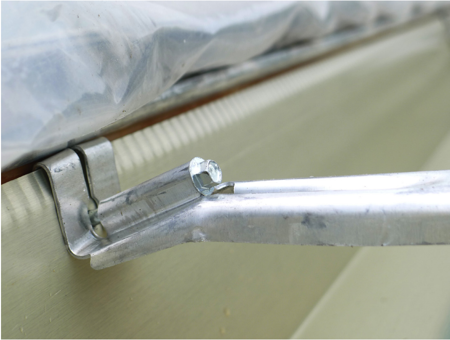
Figure 10. Professional grade gutter brackets.
