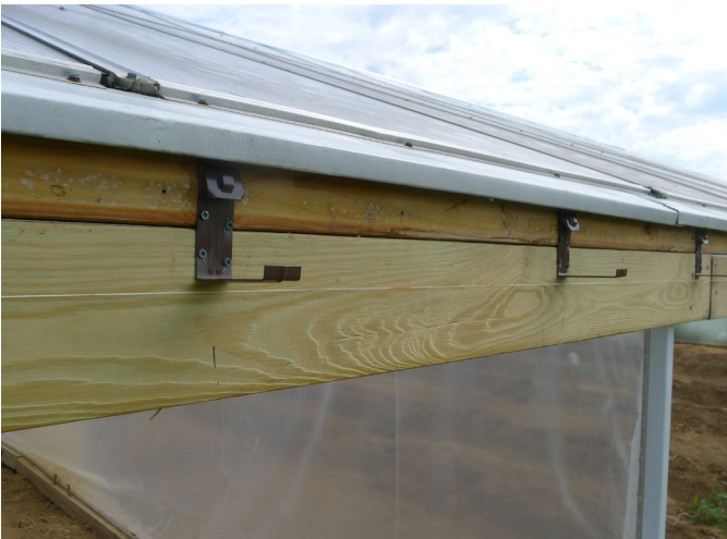
Figure 11. Gutter brackets (not recommended) for use with do-it-yourself sectional gutters.
