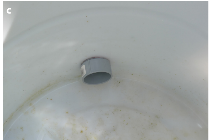
Figure 18a, b, c. Gray, 2-inch electrical conduit fittings (a) used to create a tank outlet which can be joined to standard white PVC pipe. A 2 3/8-inch hole saw was used to cut the hole in the tank (b). Different fittings are installed outside (b) and inside the tank (c).
