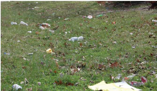
Trash and debris accumulate in a grass swale. Trash and debris should be removed after every rain of more than one inch.
