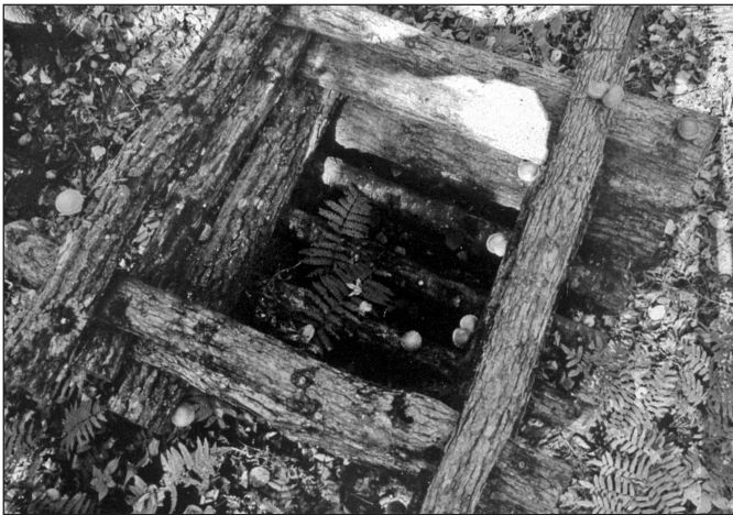
Log cabin stacking
