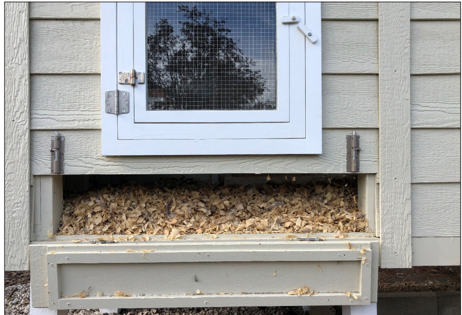
Figure 4. A cleanout door for removing deep litter from a painted plywood floor.
