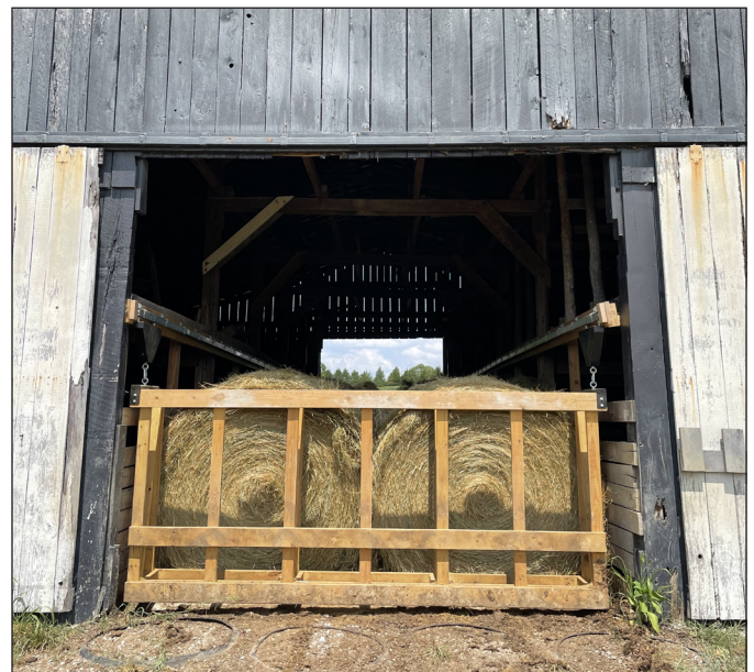
Figure 7. The southern end of the barn provides cattle access to the self-feeder with a Mechanical Concrete approach. The flooring in the barn was existing concrete.
