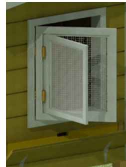
Figure 3. A dual door for the house consists of a screen and a removable glass door.
