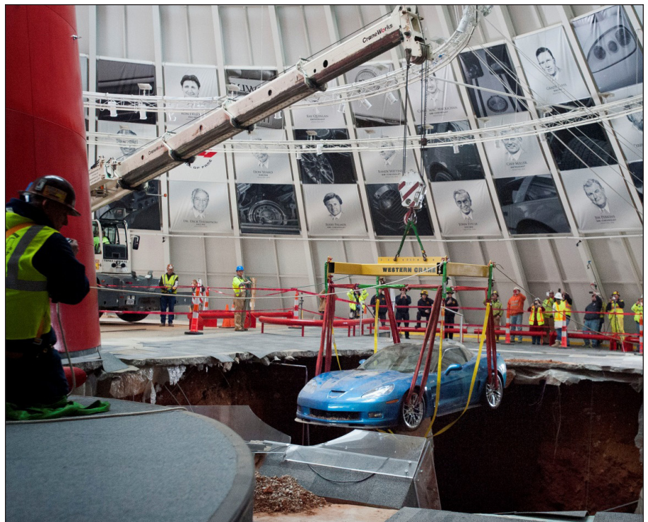
Figure 7. The February 12, 2014, sinkhole collapse in the National Corvette Museum in Bowling Green, Kentucky, is an excellent example of a cover collapse sinkhole.
