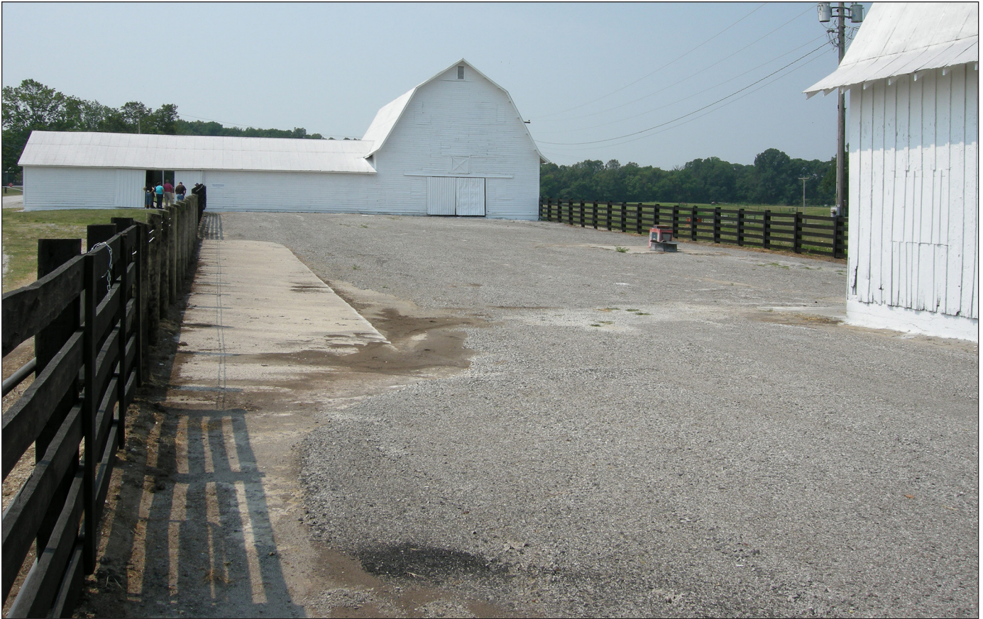
Figure 4. Example of a feeding lot using geotextile fabric and rock.
