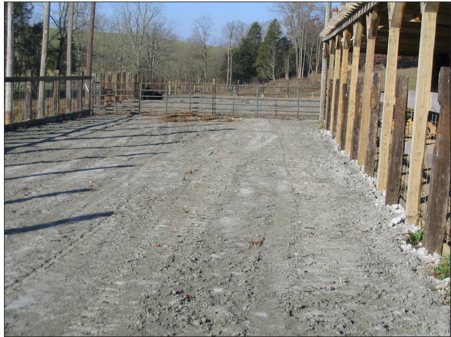
Figure 8. A cattle feeding pad constructed with coal combustion by-products.
