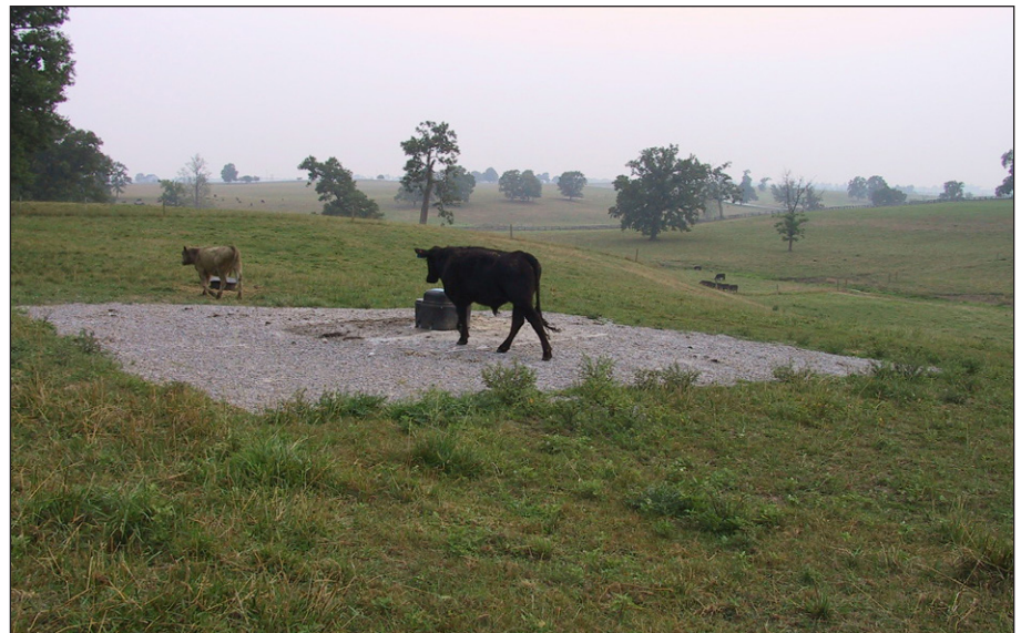
Figure 5. Adequately designed concrete pad, foundation, and heavy use area pad constructed of concrete, geotextile fabric, and rock.
