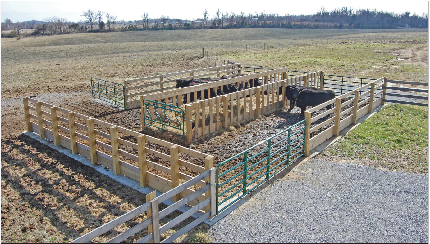
Figure 6. This picture shows two surfaces to support livestock: a concrete surface for feeding cattle and scraping and a heavy use area pad made of compacted rock and geotextile fabric.
